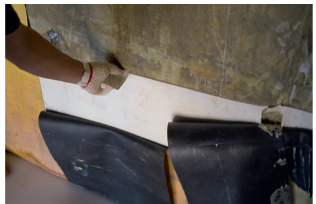
Inspection of a subsequently injected waterproofing membrane
