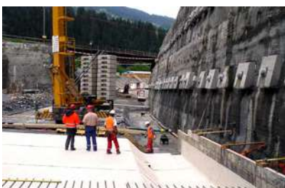
Tunnel Küblis | Switzerland
