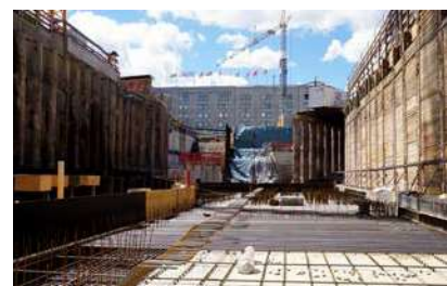
Train Station S21 Stuttgart | Germany
