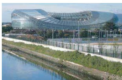
Aviva Stadium Dublin | Ireland
