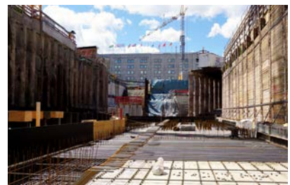
Train Station S21 Stuttgart | Germany
