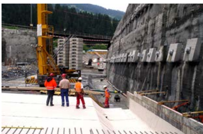
Tunnel Küblis | Switzerland
