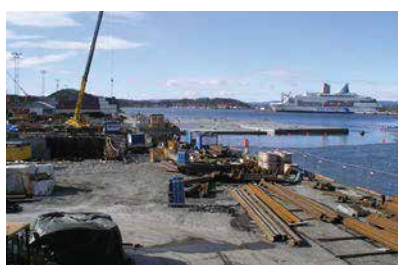
Bjrvik tunnel Oslo | Norway
