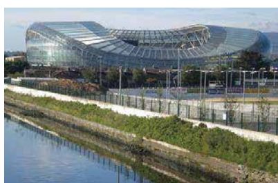
Aviva Stadium Dublin | Ireland
