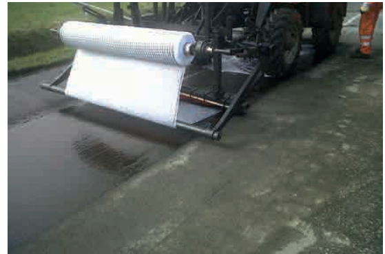
Pic. 4: Fabric Tractor Installation of GlasGrid CGL
