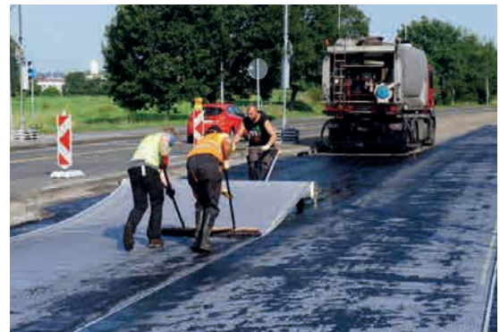
Pic. 5: Manual Installation of GlasGrid
