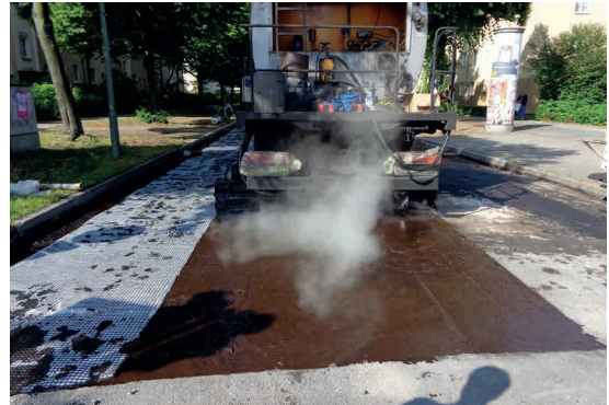
Pic. 3: Tack coat application before GlasGrid® CGL installation
