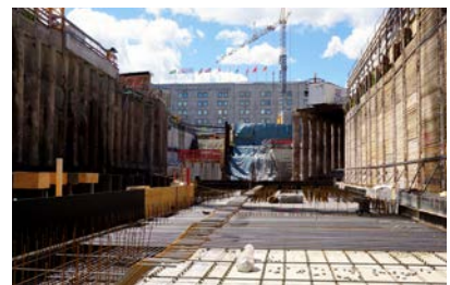
Train Station S21 Stuttgart | Germany
